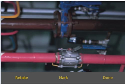
5. Point the S531 towards the leak point, and click the **Camera** icon or press the
